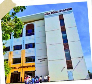
Hoa Dong Station
